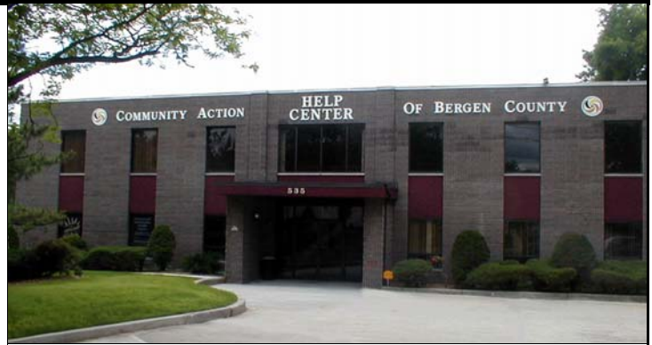
The new HELP Center in Garfield.
